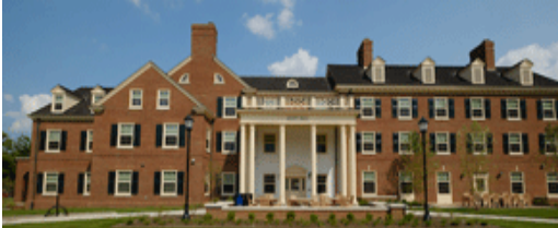
Minnich & Scott LEED Gold
