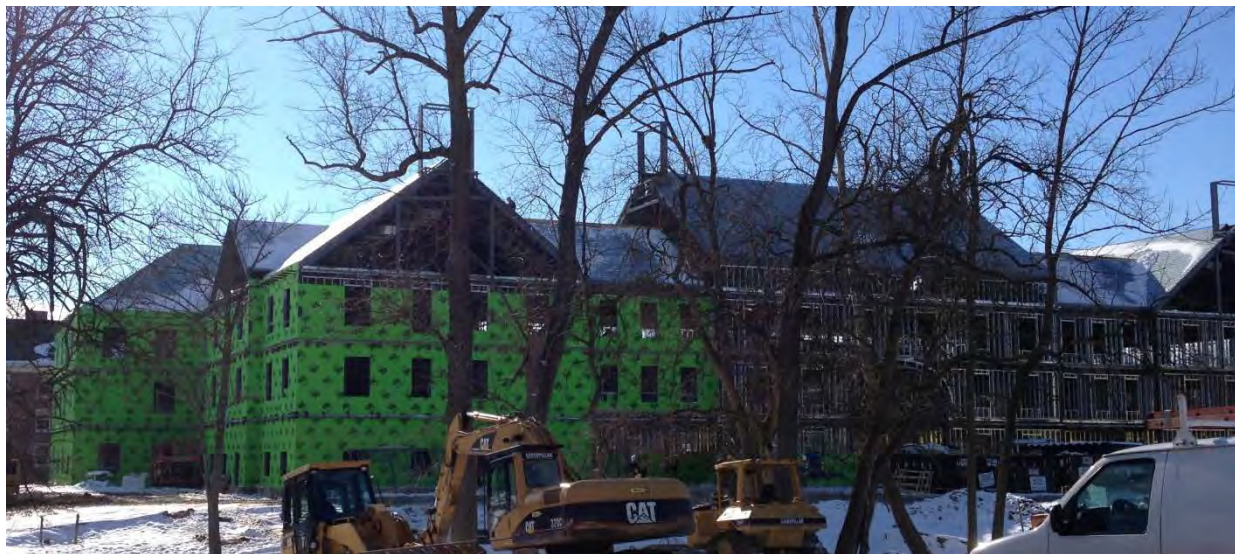
Etheridge Residence Hall Site
