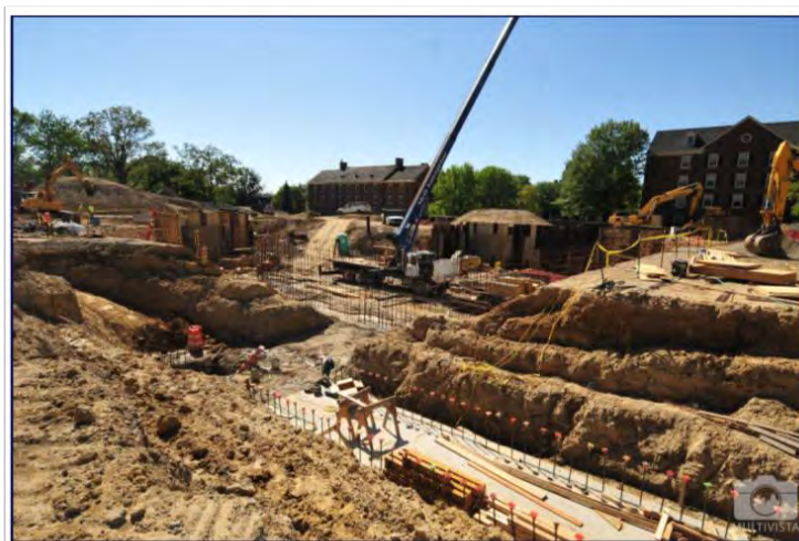
Etheridge Residence Hall Site
